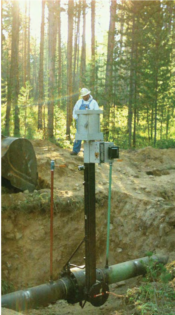
Figure 2 - Installation of Becker Below Ground Ball Valve Regulator.
